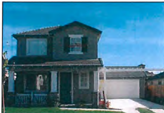
b) Richly detailed surfaces, modulated facades and varied roofline create attractive, street-facing facade.
