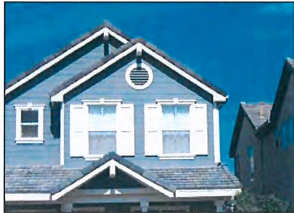
a) Varied roof planes and second story facade details add visual interest.
